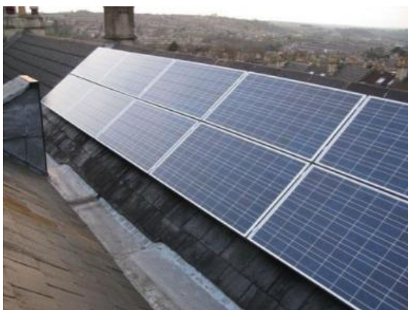
Southerly Facing Solar Panels inside the pitched-roofs of Listed Buildings.
