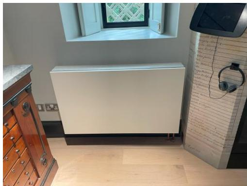
A bespoke fan heater powered by the heat pumps has been installed at the base of the tower to preserve the fabric of the tower:
