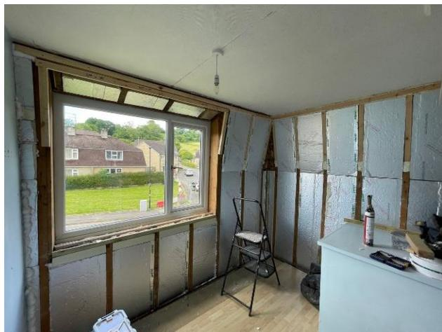
This work should have halved heat losses from the walls on the first floor. It's important when fitting Celotex like this to install it tight on the timber frames to avoid thermal bypass. Guy is planning to insulate his home's mansard roof in the future.
