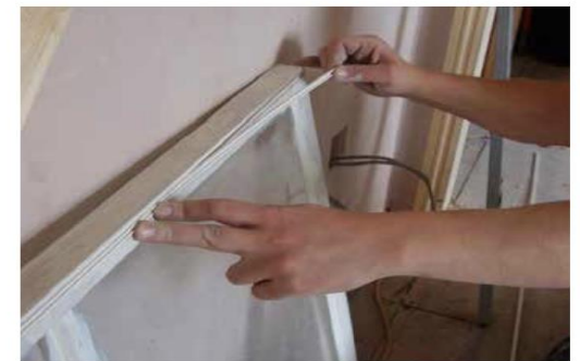
Figure 8 (top) Brush pile seals added to a sash window.
